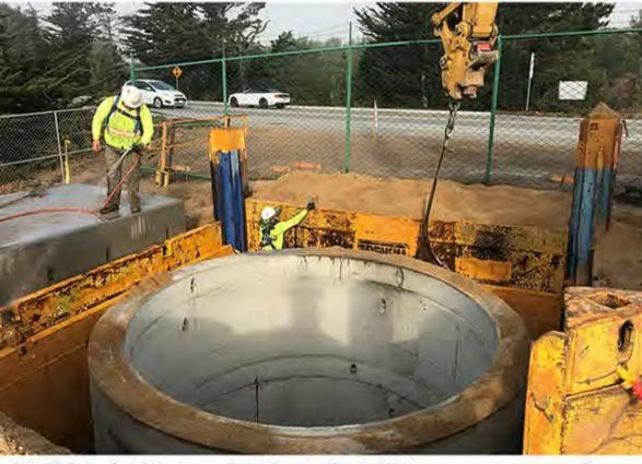
Imjin Lift Station Capital Improvement Project: Crews installing the 12' diameter precast concrete wet well.
